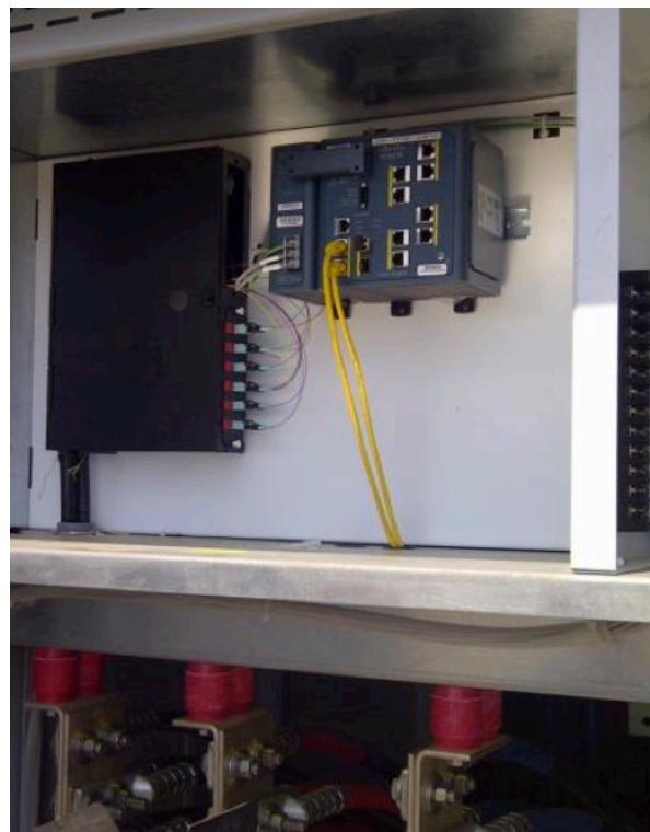
Terminal Monitoring Data monitoring di Panel Kontrol. Sumber: Triad Engineering. Foto: Dan Jordan
