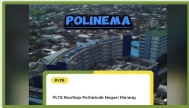
Rooftop Solar Panel
